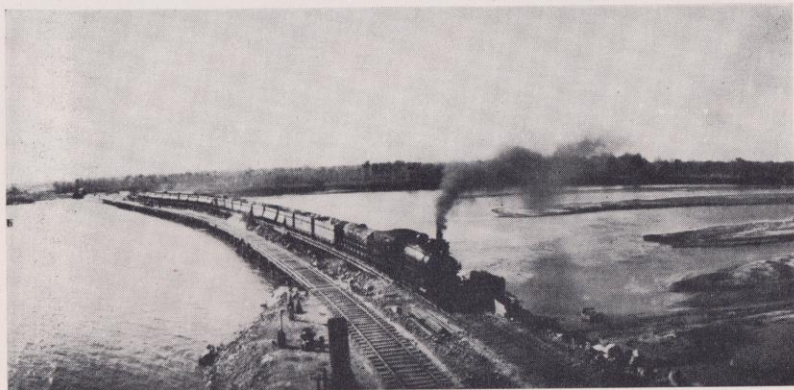
Rocks were hauled to close the widening gap.
